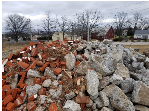
The Hickory Grove One-room School, above and now recently demolished.
